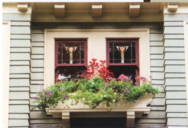
The 1911 exterior is marvelously detailed, with novelty siding, exaggerated columns on piers, leaded and stained glass, brackets—and now a great color scheme.
